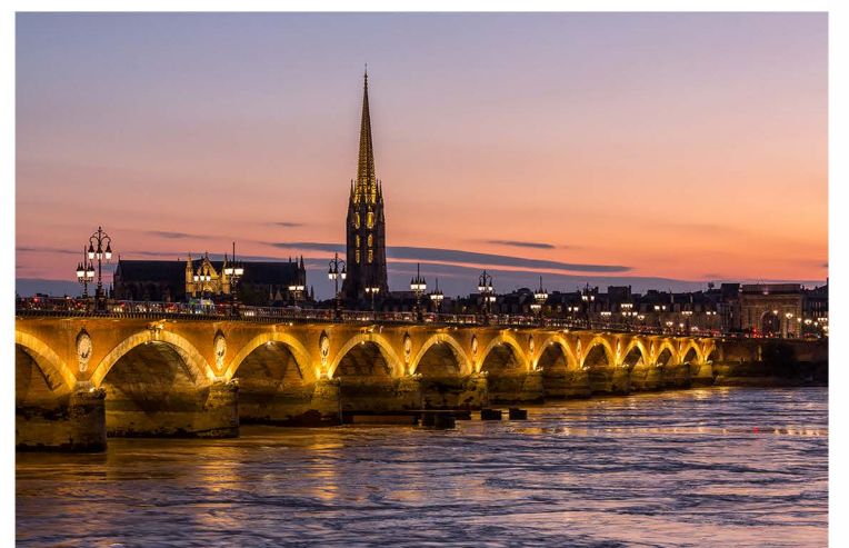
Bordeaux: Pont de pierre (Stone bridge) Credit: Steve Le Clech
